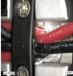
Incorrect Placement (Strap bowing and pinching wires)
