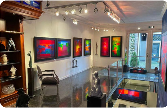
Old lighting before renovation.
